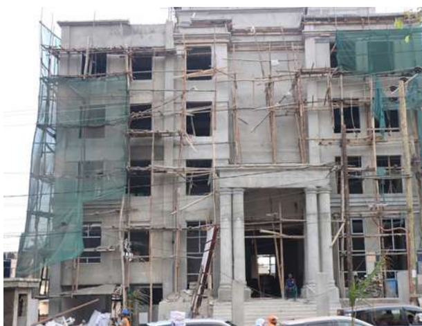
Front view of the ULS House as of June 2024
