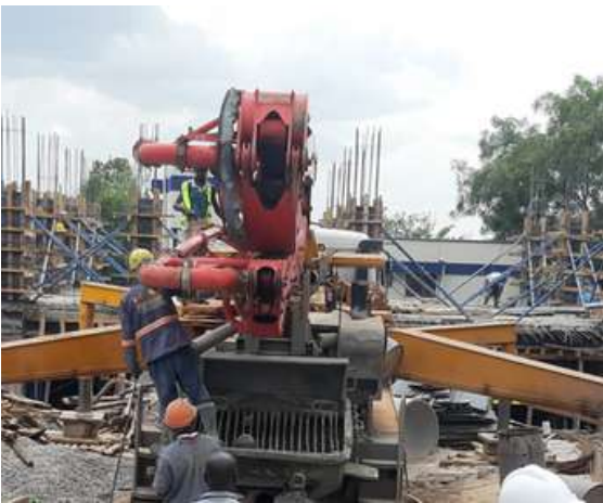
Excavation and ground breaking works
